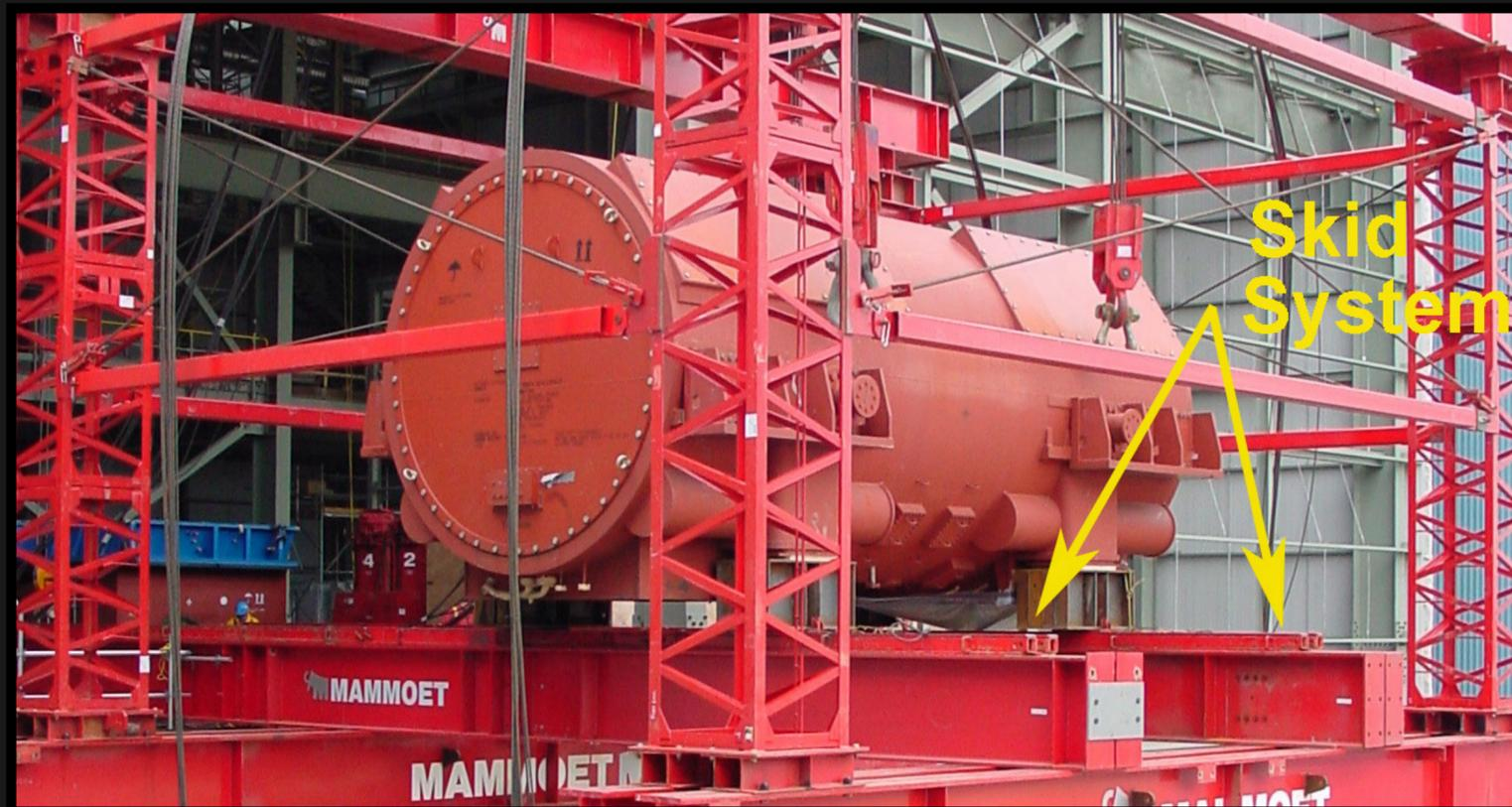
Installing a generator at height using a Skid System and Strand Jack Tower combination
