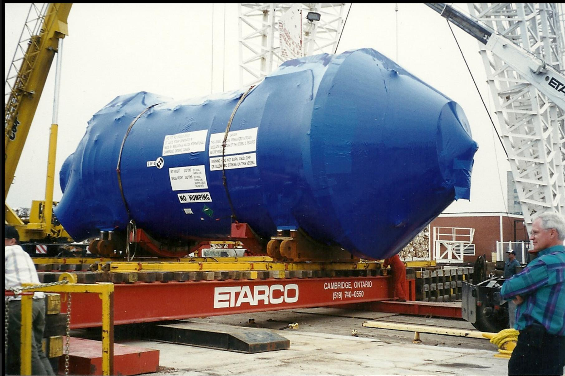
Loading a Steam Generator onto a free floating barge with a skid system
