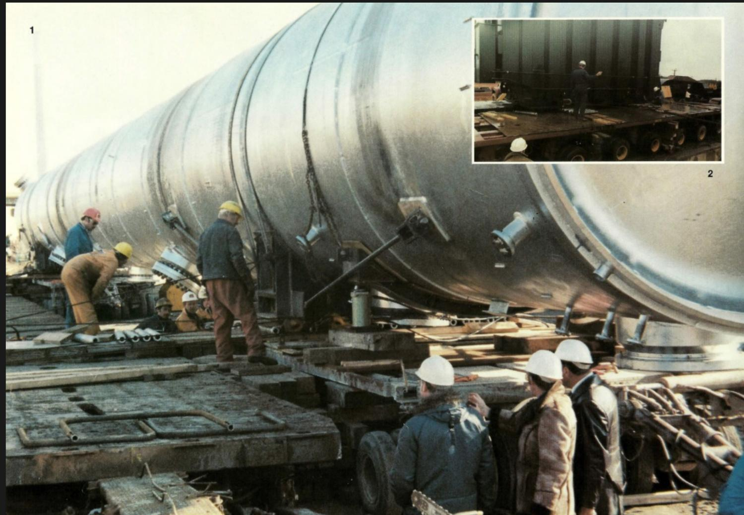
**Unguided System: No restraints to stop the load from moving in unwanted directions.**
